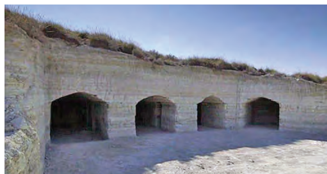
The tunnels before work started
